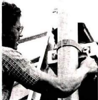
Mounting the House Bracket
