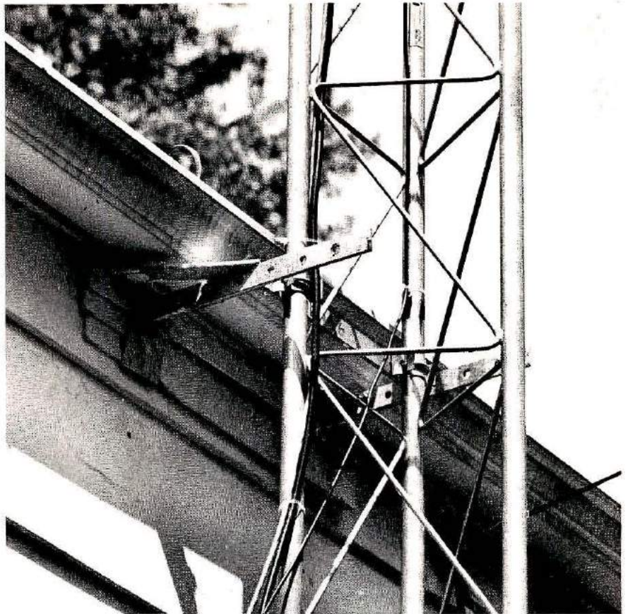
A bracket to hold the tower to the house will take the place of guy wires — up to a modest height, at least. The brackets are adjustable, but some wood shims were needed to be sure the tower was exactly plumb.
