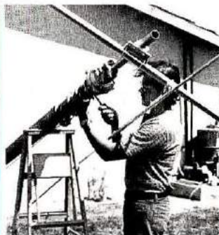
The Hinged Base Plate allows tower to be tilted over for access to antenna and rotor from the ground.
